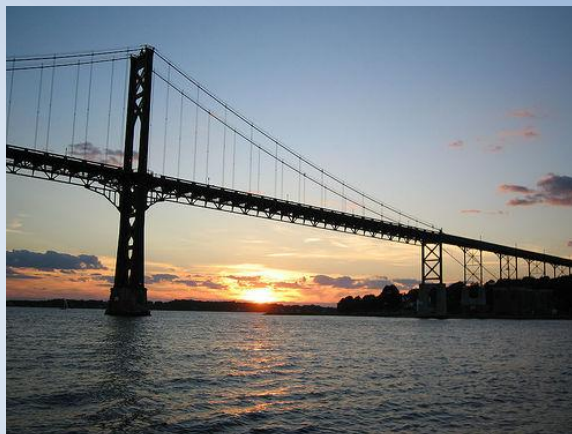
Bridge in Mt. Hope Bay from Bristol to Portsmouth. RI
