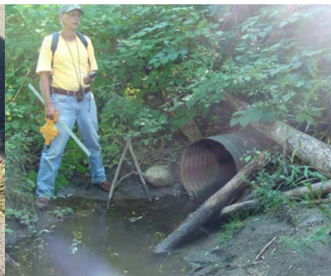
Stormwater Outfall from Madison Ave.
