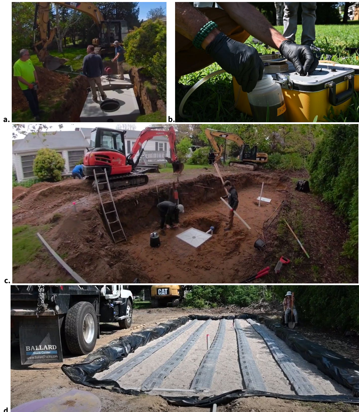
Figure 8. Screenshots of experimental Layered Soil Treatment Area septic system installations in Charlestown, Rhode Island. Four systems are being installed under an EPA Southeast New England (SNEP) funded pilot project. This is a non-proprietary system with design features allowing easy performance monitoring and inspection. A. standard septic tank b. effluent sample collection to measure nitrogen concentration; c. excavation for disposal field showing pan lysimeters which facilitate monitoring; d. pressurized shallow drainfield (PSD). Source: Video by the Town of Charlestown, available at https://www.youtube.com/watch?v=KJ6oGT1VaU8 .
