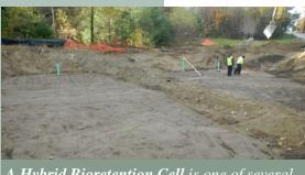
A Hybrid Bioretention Cell is one of several BMPs currently being installed at Russell Rd. in Skowhegan. Photo: Acorn Engineering
