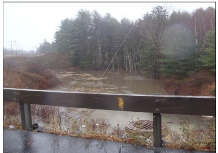
Figure 12: Stormwater detained behind the Midway Drive road crossing. (C. Rinehart, Wright-Pierce).
